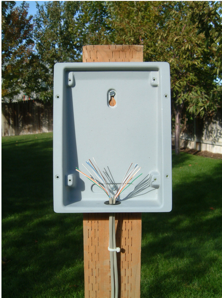
Figure 3 - Mounting the enclosure
